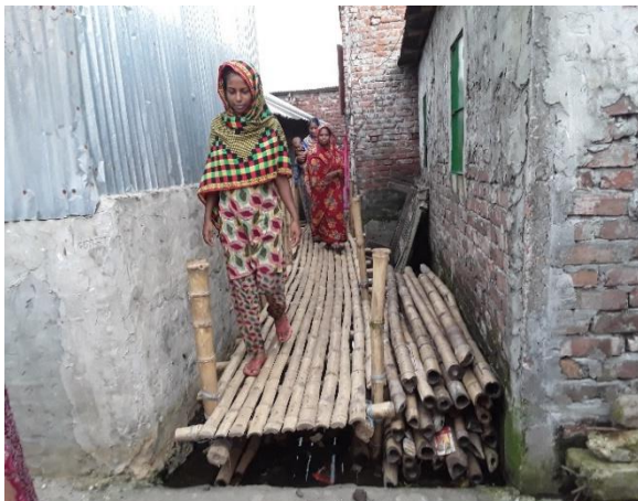
Temporary Elevated Path Using Bamboo
