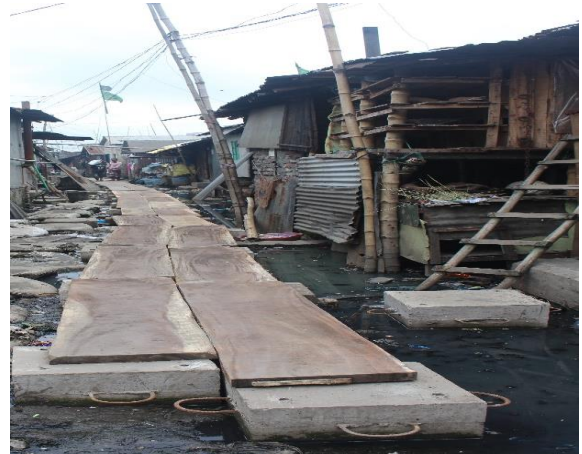
Temporary Elevated Path Using Concrete Blocks
