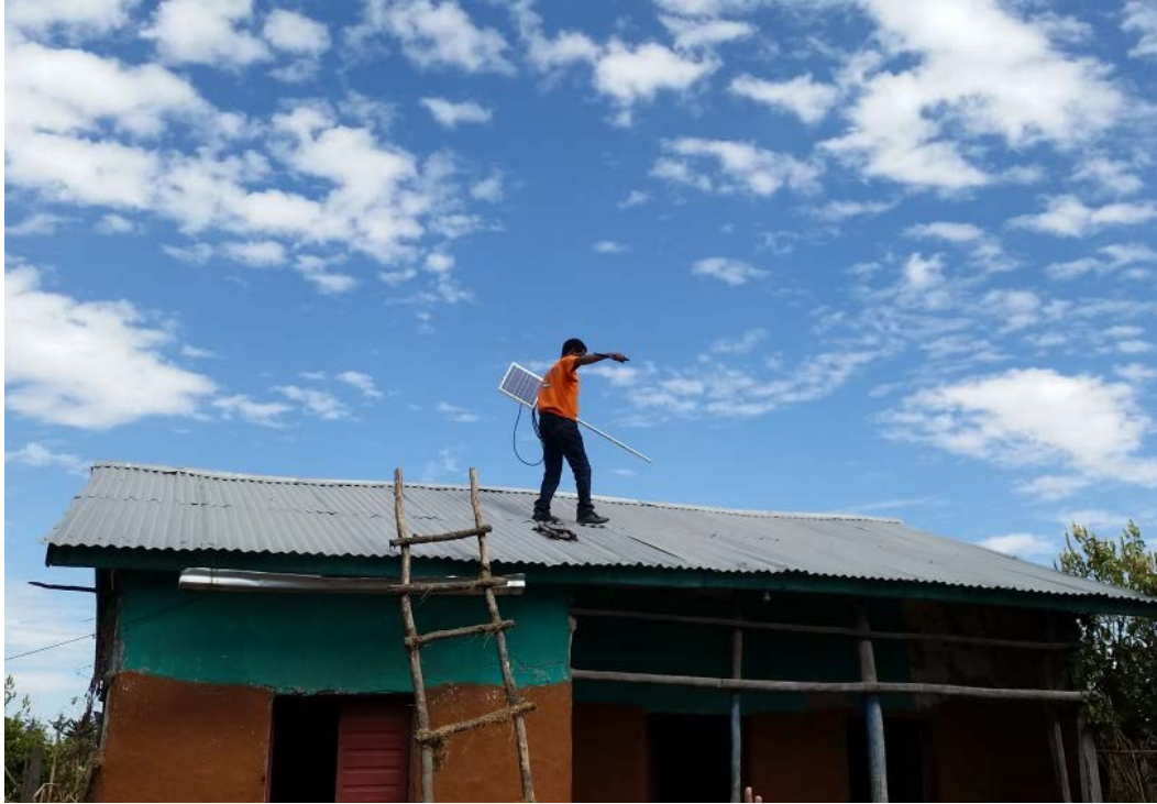
Figure 1. Installation of a solar home system by a staff member of a CET provider. Copyright: Gaia Consulting Oy
