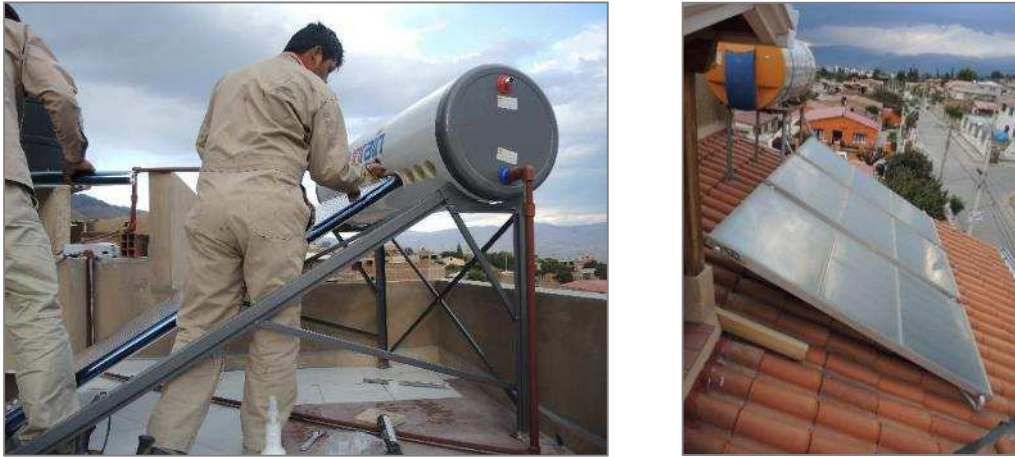
Figure A3.1: Installation of solar water heater and Installed Solar Water Heater
