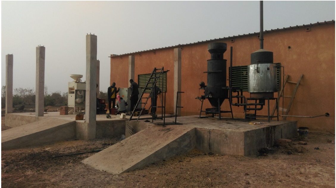
Figure 21 Installation platform for gasifier and genset
