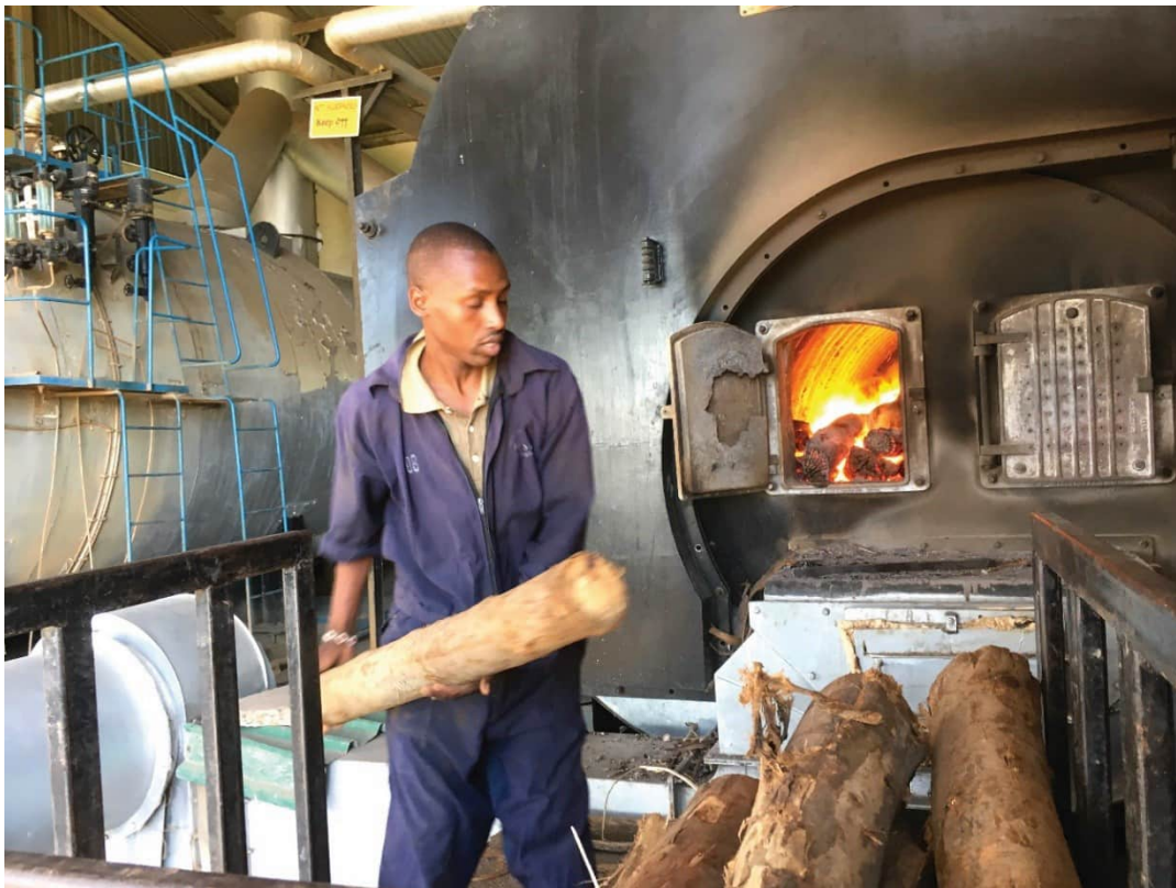
Firewood boiler at Chelal tea factory. Photo: Absolicon
