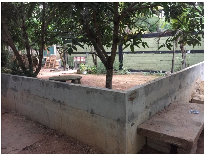
Picture 5 New wall built in Gampaha SME unit to block flood waters
