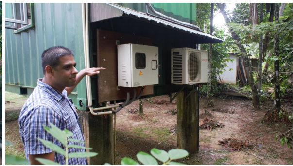
A local herb tea producer lift its workshop and equipment to reduce flood losses
