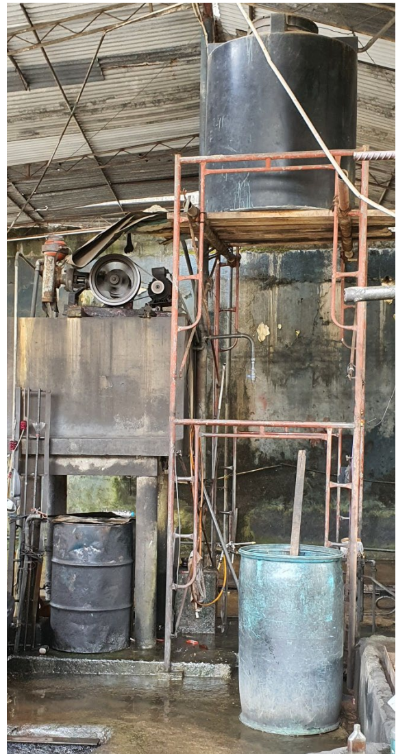
Local manufactories' generator and pump raised above ground/flood level to avoid flood damages
