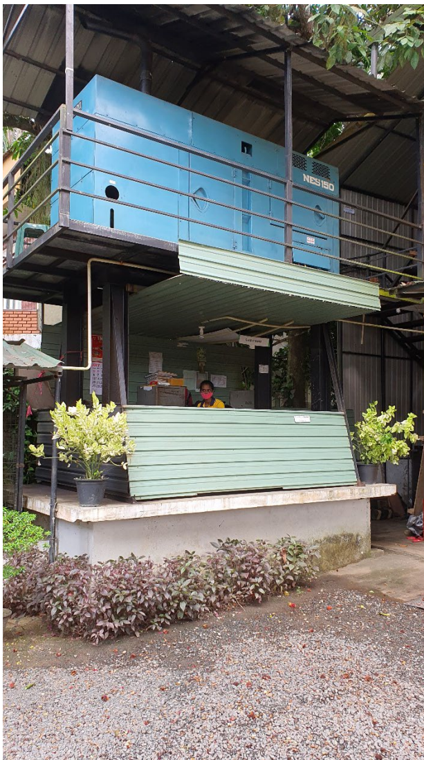
Local manufactories' generator and pump raised above ground/flood level to avoid flood damages
