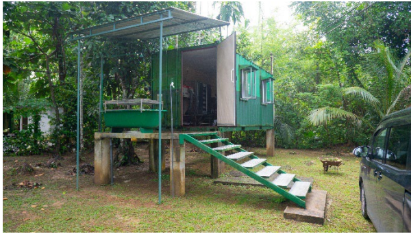
A local herb tea producer lift its workshop and equipment to reduce flood losses
